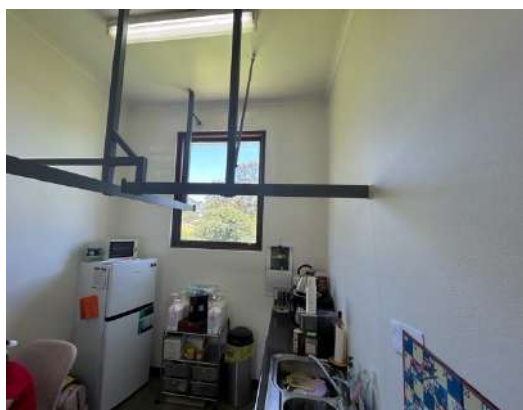
Image shows room to the rear of the property, with timber framed window and concrete floor as well as rails used as part of the buildings former use as a butcher shop.
